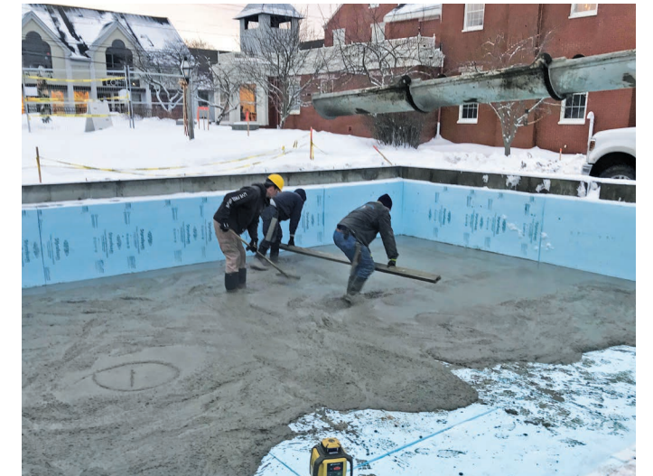
Photo 6: Floating the new slab
