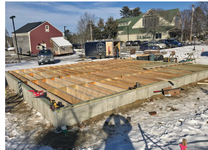
Photo 7: New wood frame floor system
