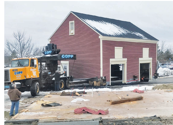
Photo 5: Barn moving off the old floor system
