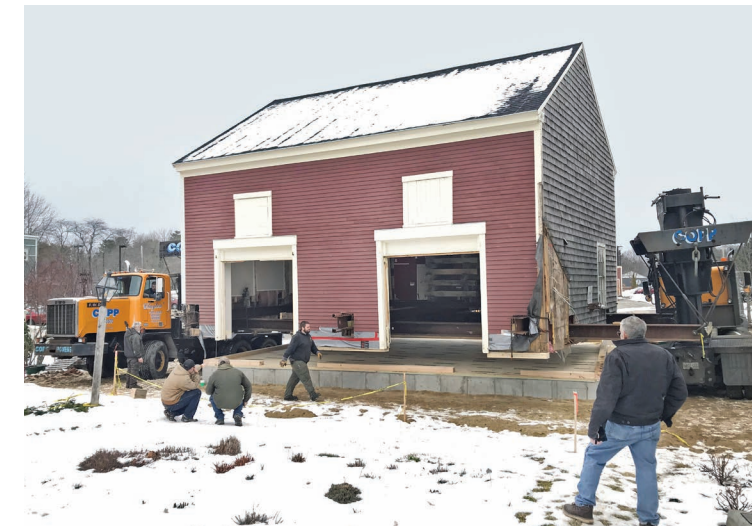
Photo 8: Barn coming down on new foundation
