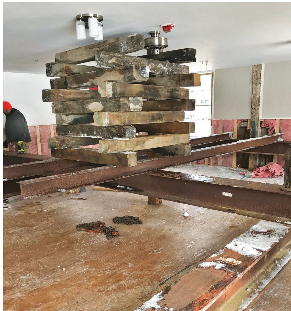
Photo 4: Interior steel & dunnage
