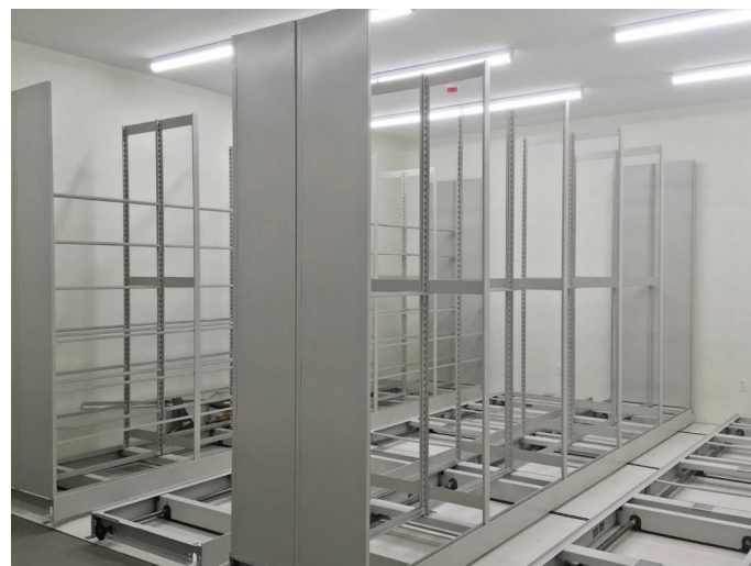
3 - The first uprights are installed.
