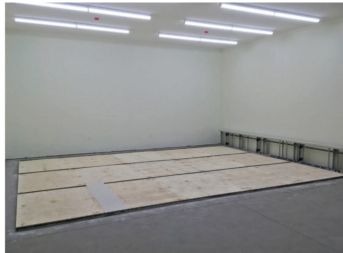
2 - Flooring is installed flush to the rails.
