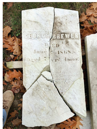
George Brewer's stone was in multiple pieces. His tablet was broken at the base, but thankfully the base was still usable, and most pieces could be located. After some very careful epoxy work and a lot of back filling George's headstone has been preserved to stand alongside those of his family members.
