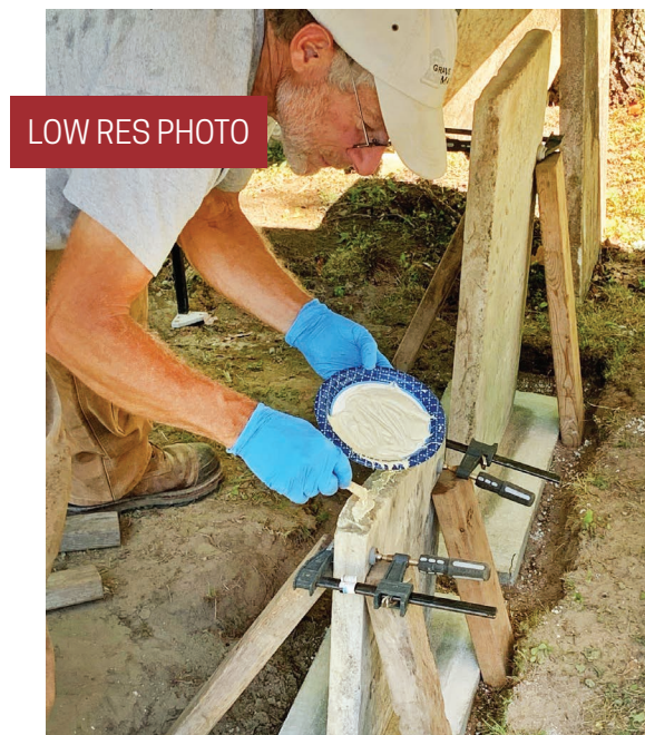
Joe Ferrannini of Grave Stone Matters set two of the Coffin family stones in new bases and used epoxy to repair fractures. Stones were then left with supports and covered to allow the materials to cure before they stand upright on their own once again.
