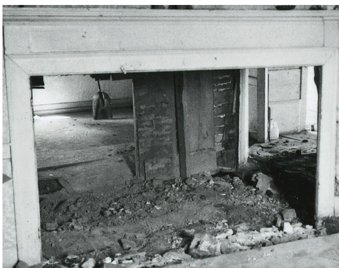
In summer 1978, the original chimney and fireplaces were dismantled and salvageable bricks were set aside.
