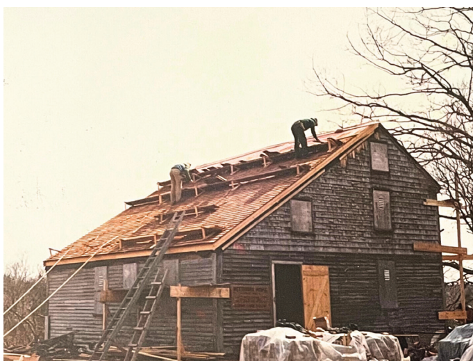
In 1980, a new red cedar roof was installed, helping to protect the farmhouse from ongoing water damage and structural deterioration. It marked a critical step in stabilizing the building and extending its life. FHS INSTITUTIONAL FILES
